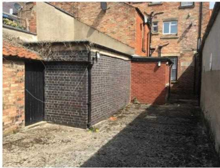
Rear Vault Extension and Toilet Block
